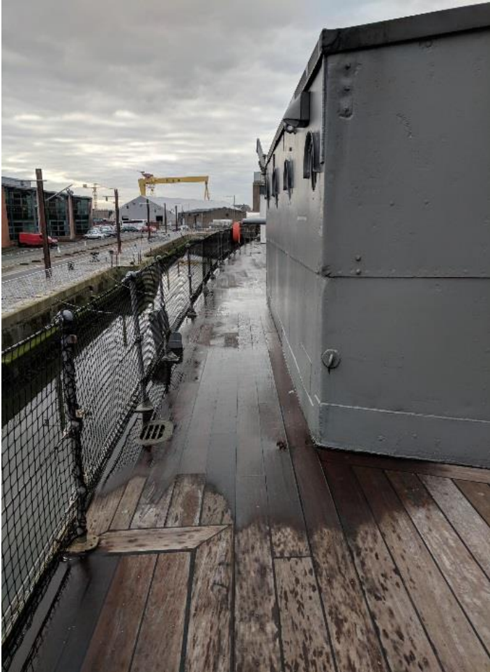
Accessible route past the Captain's Quarters
