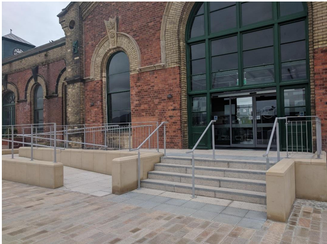
Pump House entrance
